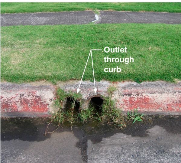
Underground pipes convey runoff to the gutter through the curb.
