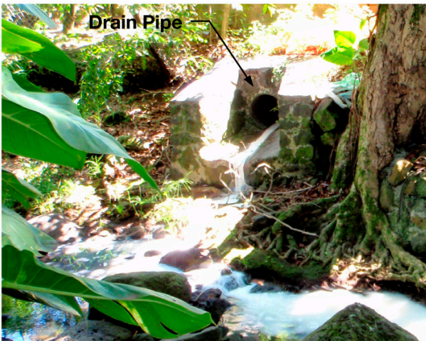
A drain pipe discharges pollutants into the stream.
