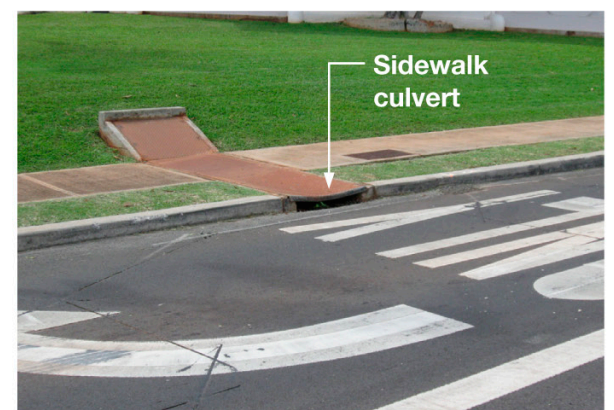
Runoff from private property is conveyed to the gutter through an opening in the sidewalk.
