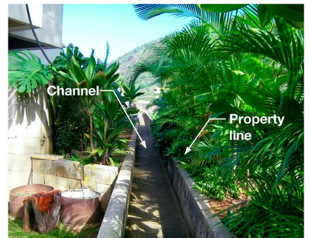
Similar to a swale, a channel within private property is a private drainage system. Each property owner of a private drainage system that ultimately connects to the City's drainage system is required to have a drainage connection license.
