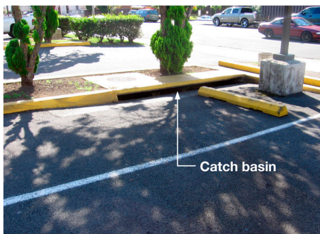
A catch basin in a private parking lot collects and conveys runoff into the City's storm drainage system.
