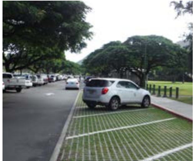
Figure 4.10: Hybrid Parking Lot (Honolulu, HI)
