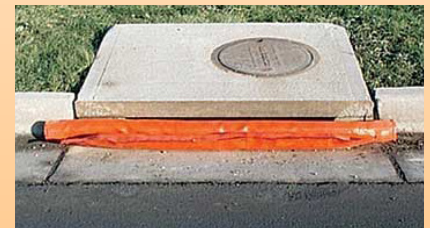
Curb inlet filter/barrier
