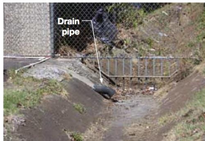
A drain pipe connects runoff from a parking lot directly into a City drainage channel.
