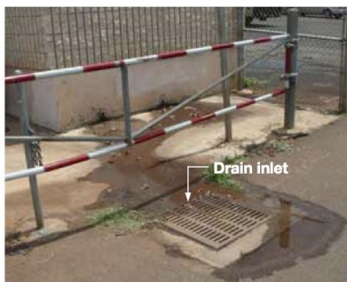
A drain inlet on a private road collects and conveys runoff into the City's storm drainage system.
