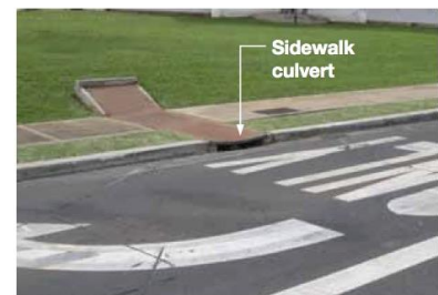
Runoff from private property is conveyed to the gutter through an opening in the sidewalk.
