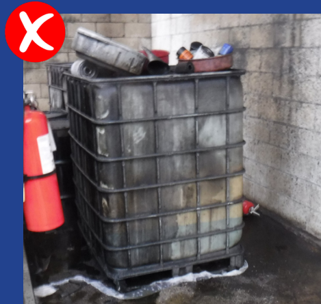
Uncovered oil container with no secondary containment.
