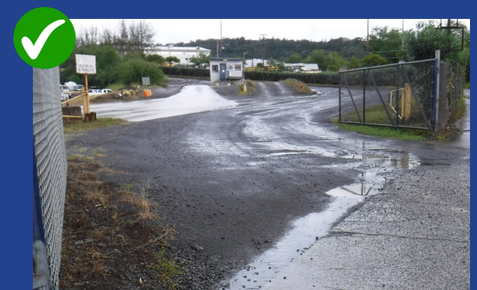
Pave or use gravel for areas where vehicles regularly travel.
