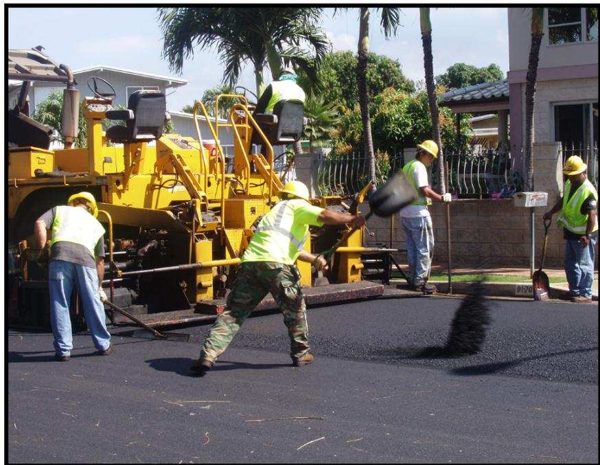
*A road repair crew applies first-aid repairs on Kilaha Street in Ewa Beach. Temporary first-aid repairs increased 291 percent between FY2001-02 and FY2003-04, while road resurfacing decreased 52 percent during the same period. Office of the City Auditor photograph.*
