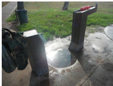
Poor drainage at Kea'au Beach Park
