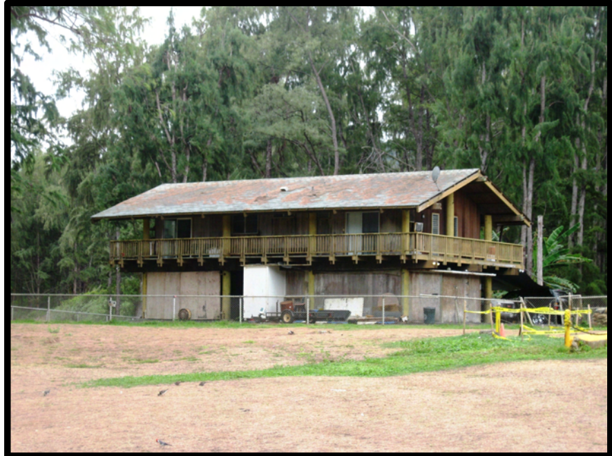
This three-bedroom, two-bath home is provided to a city employee in exchange for enhanced on-site services at Waimanalo Bay Beach Park.
