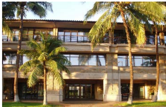
James Campbell Building
