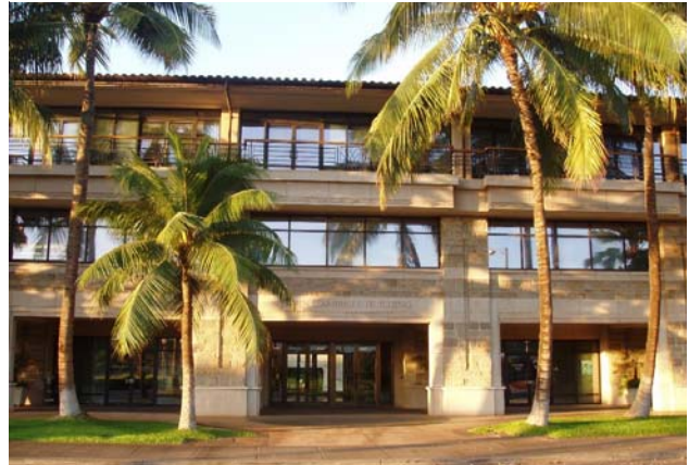
James Campbell Building
