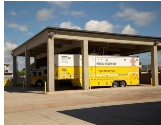
East Kapolei's Regional Emergency Depot houses emergency supplies and equipment that can be deployed to a long-term, large-scale emergency or to fire stations on the Leeward Coast that might be affected or become isolated during a disaster.
