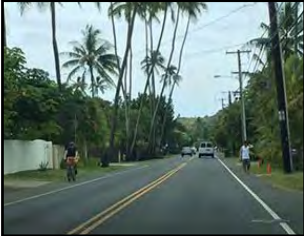
Kalaheo Avenue Shoulder Improvements
