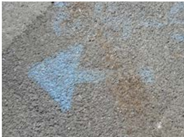
Markings to Identify Meter Locations
