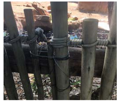
Exhibit railing fastened with various wires/ropes
