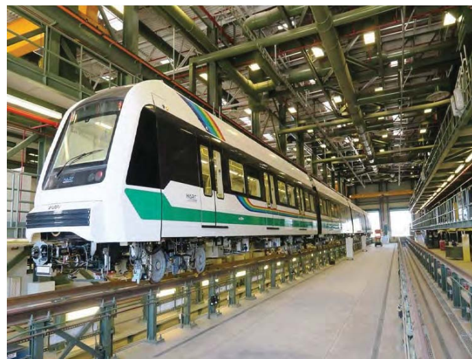
HART Maintenance and Storage Facility
