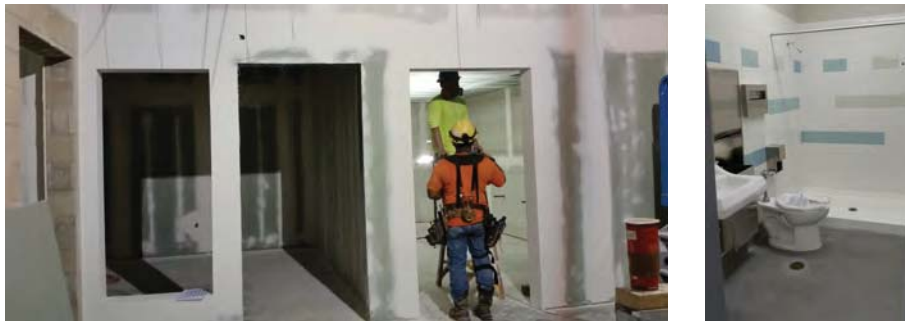
Pūnā wai Rest Stop (Under Construction)
