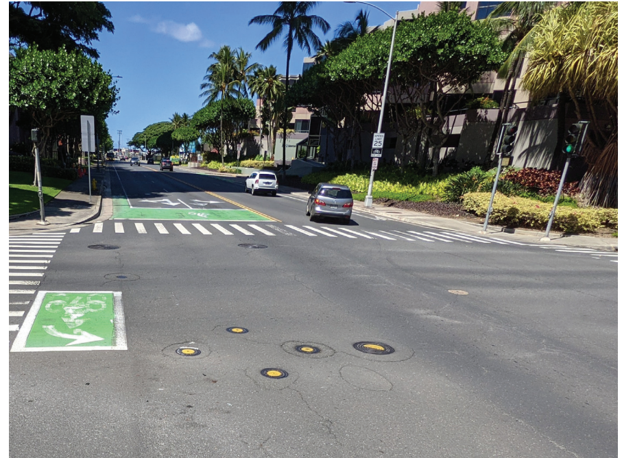
Example of a two-stage turn queue box on the intersection of South Street and Pohukaina Street.
