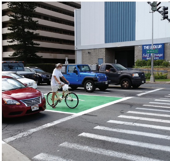
Bike box on intersection of McCully St. and Kapiolani Blvd.
