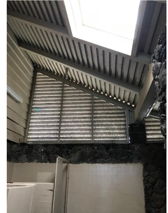
Louvered Windows + CMU Walls
