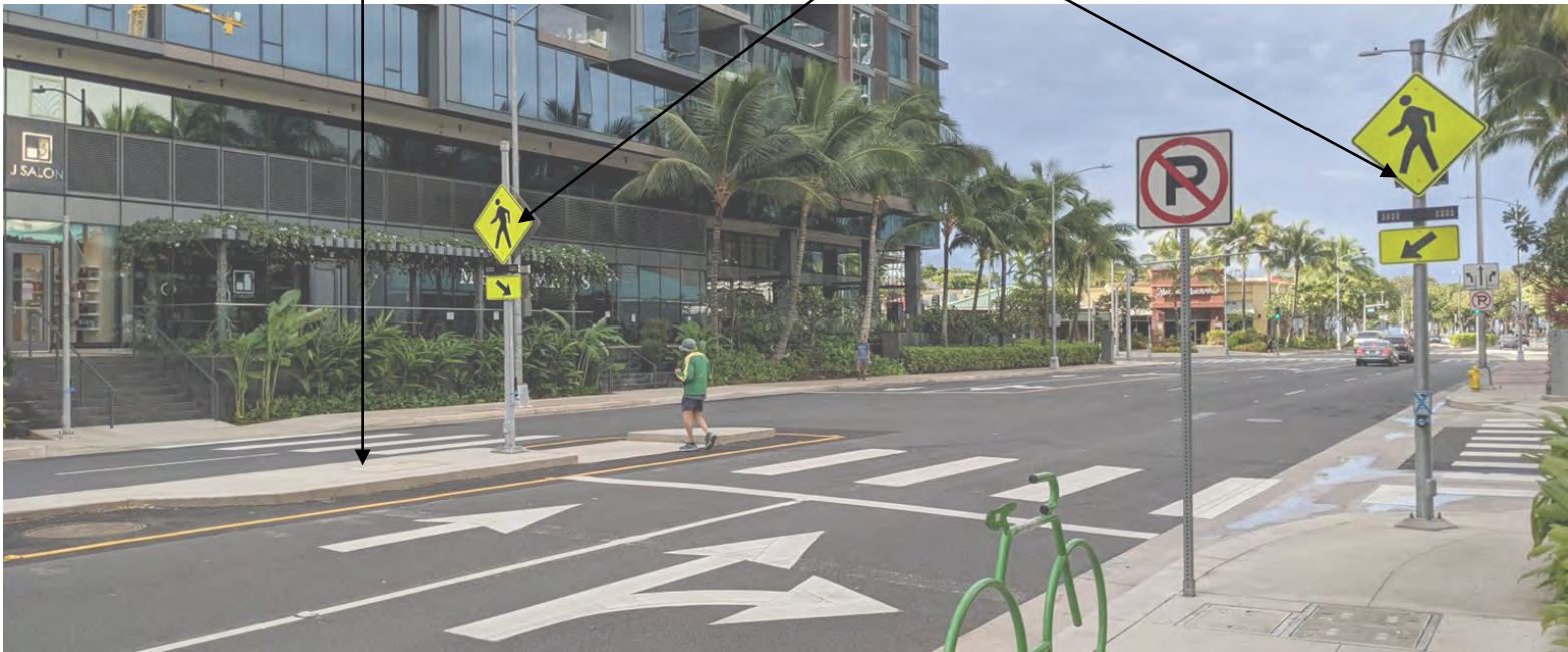
RRFB crossing with a median refuge island, Kamake'e St.
